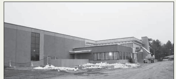
East Building elevation looking south-southeast, March 22, 2022
